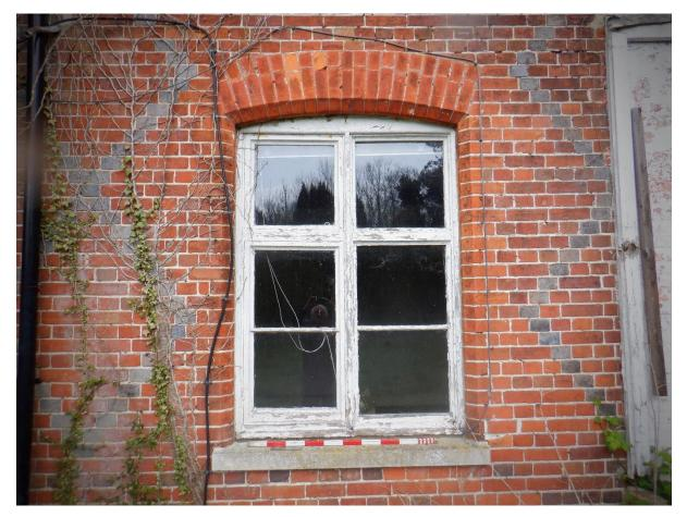
Plate 8. Detail of external wall and casement window (1m scale)
