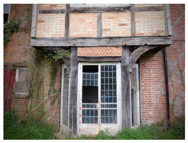
Plate 12. Detail of timber framed extension on NE façade (1m scale)
