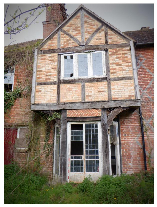
Plate 13. View of timber framed two storey timber framed bay extension
